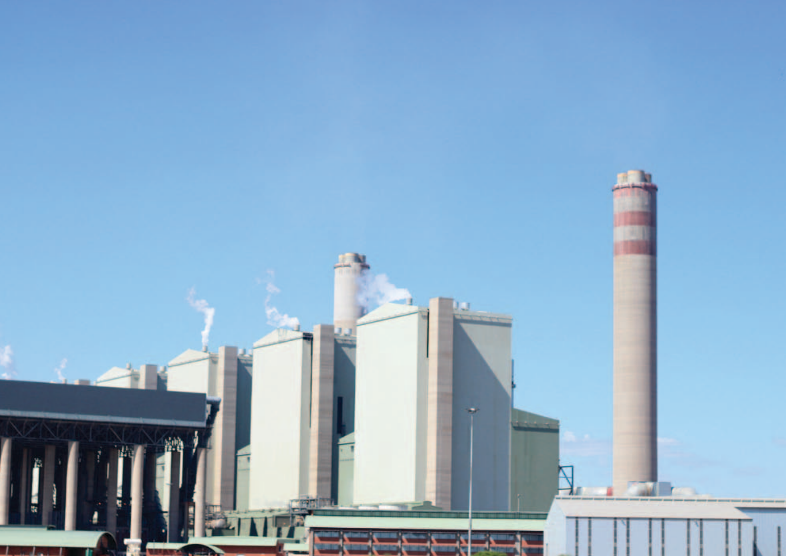
Medupi Coal-Fired Power Station, Lephalale, Limpopo province.
